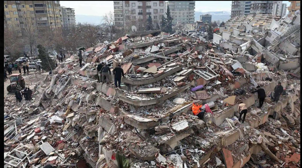
Collapsed buildings in Kahramanmaraş, Türkiye.
